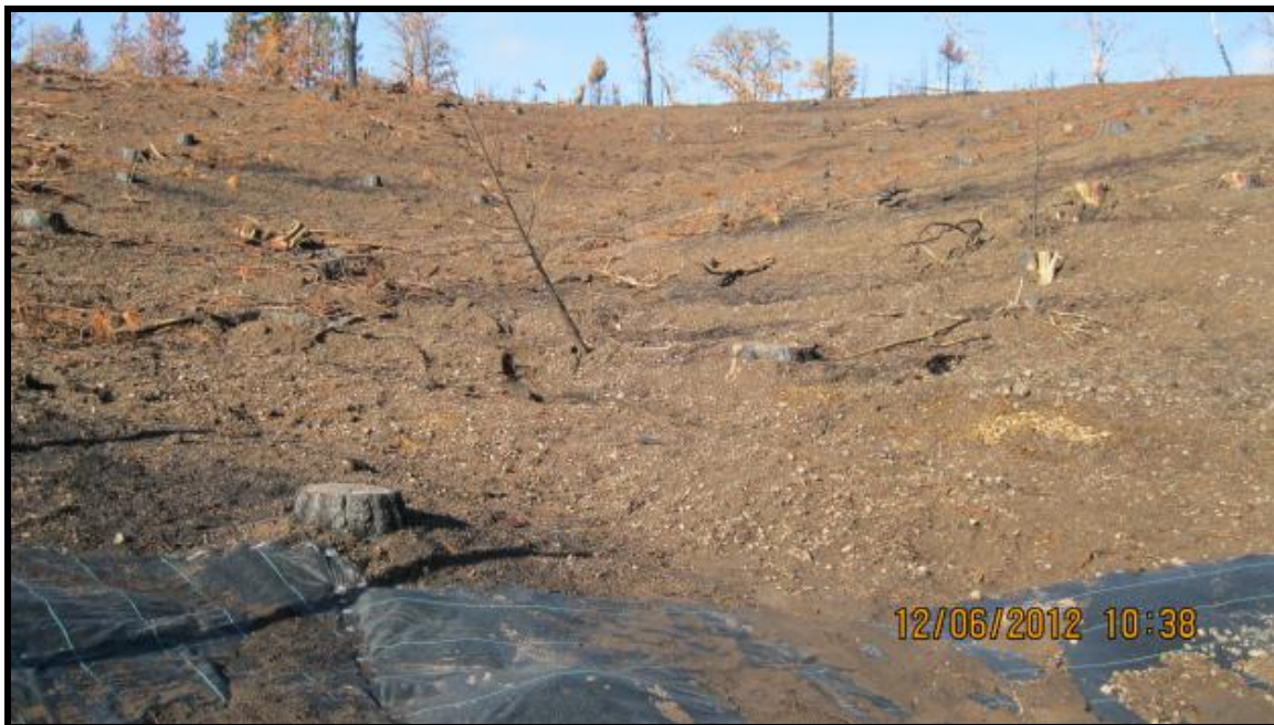
Figure 34. Contour ripped swale above fence #1.
