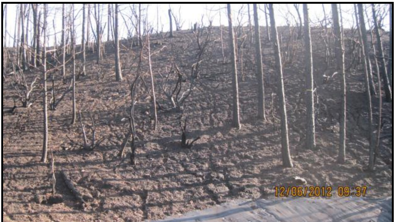
Figure 10. Rill erosion above fence #8
