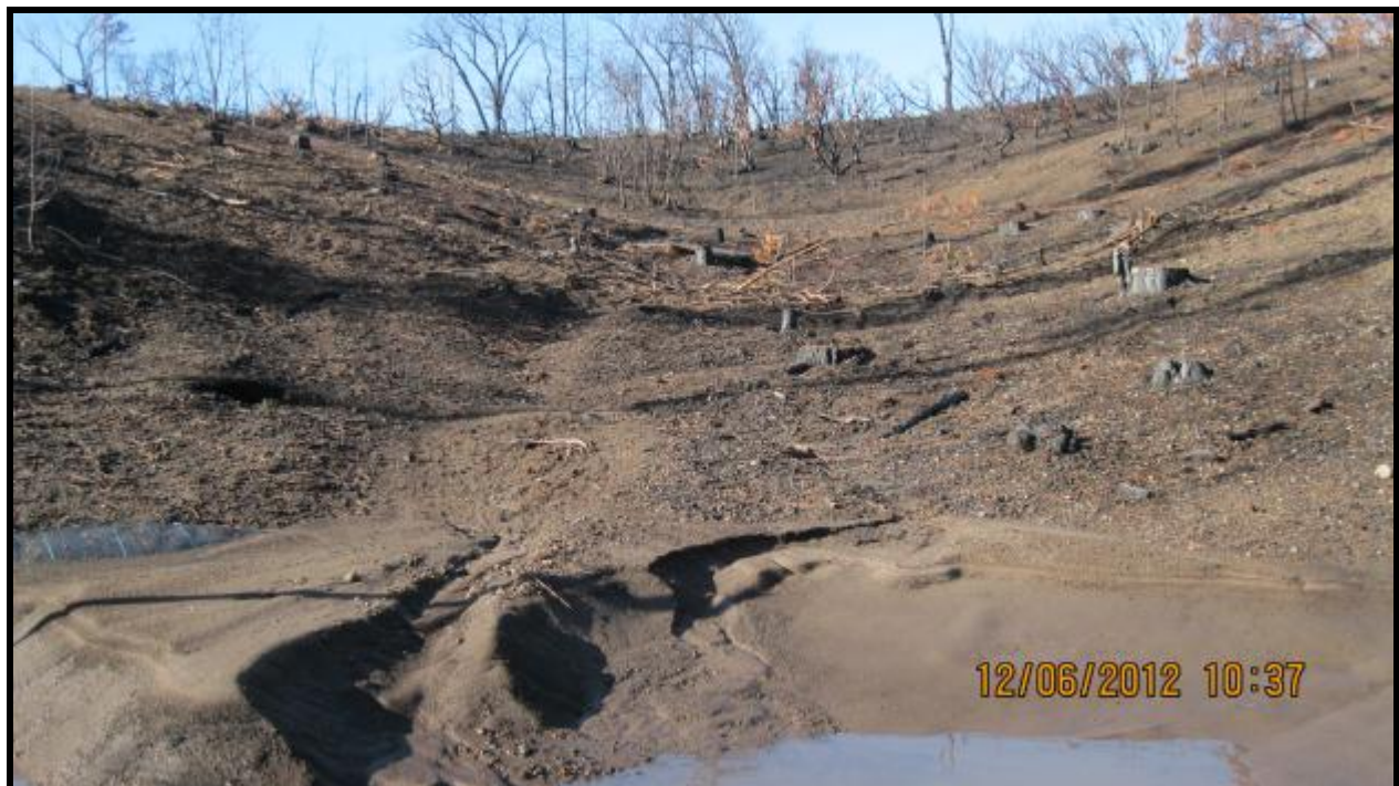
Figure 32. The lower portion of the swale draining to fence #2.
