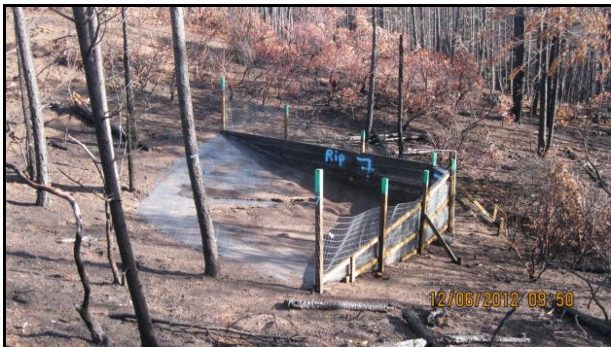
Figure 13. Sediment deposition in fence #7.
