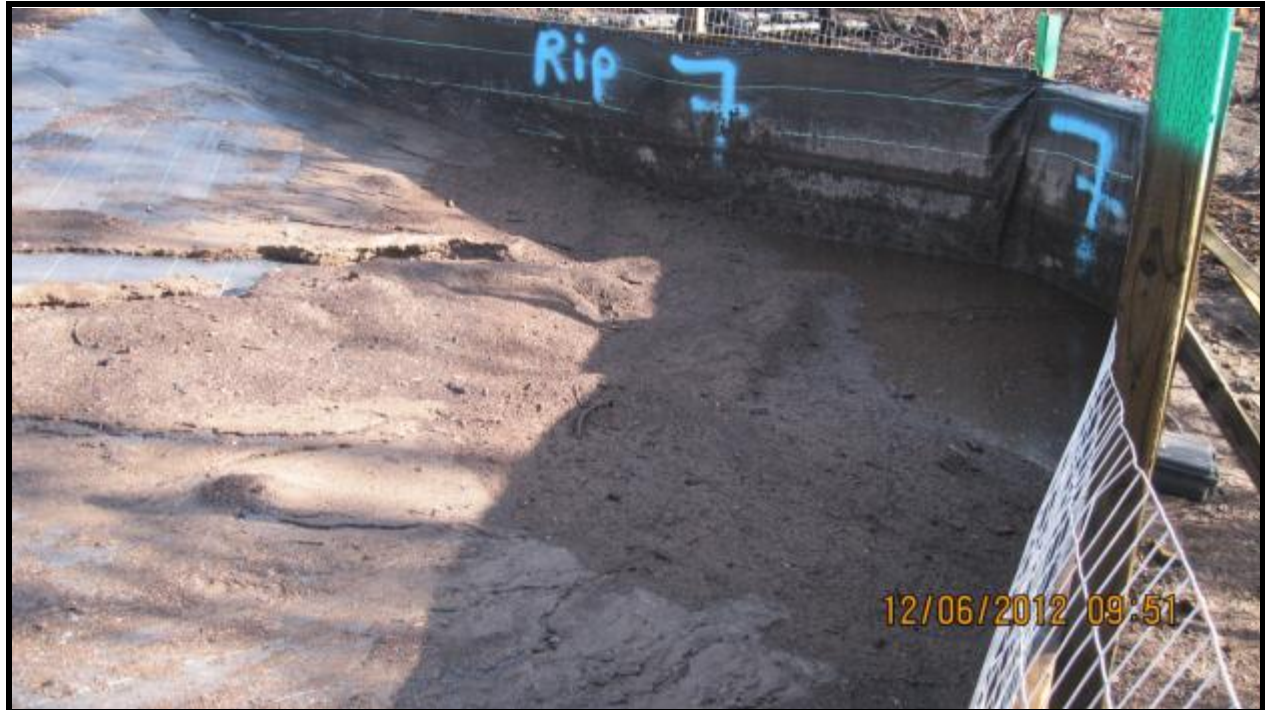
Figure 14. Sediment deposition in fence #7.
