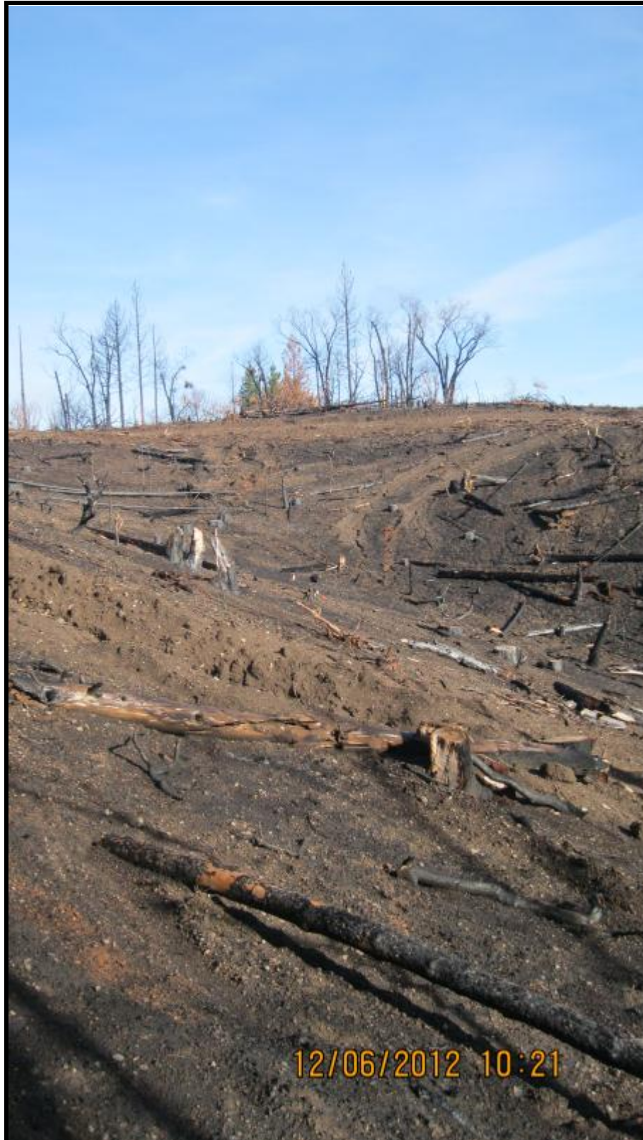
Figure 25. Equipment tracks on the upper portion of the swale draining to fence #4.
