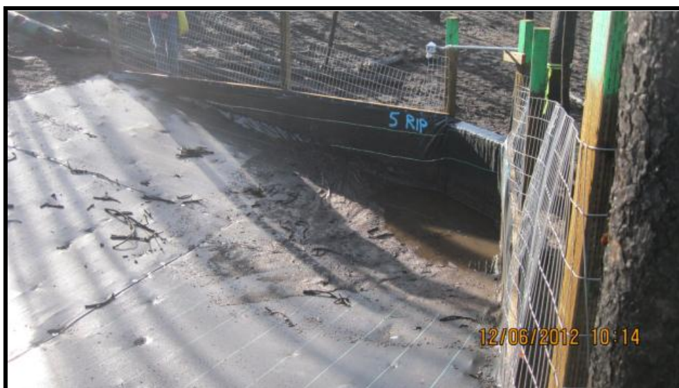
Figure 21. Deposited sediment in fence #5.
