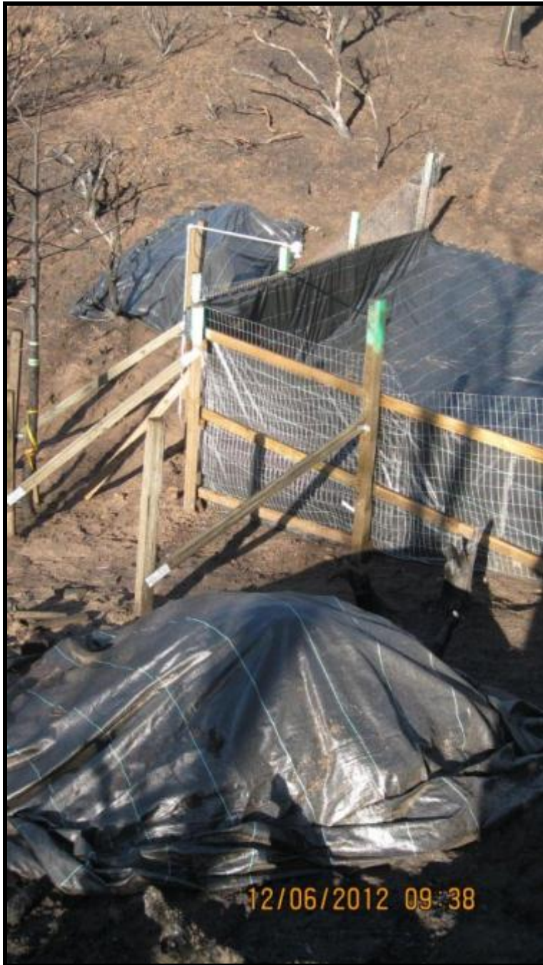
Figure 8. Excavated material from fence #8 wrapped in sediment fence fabric.
