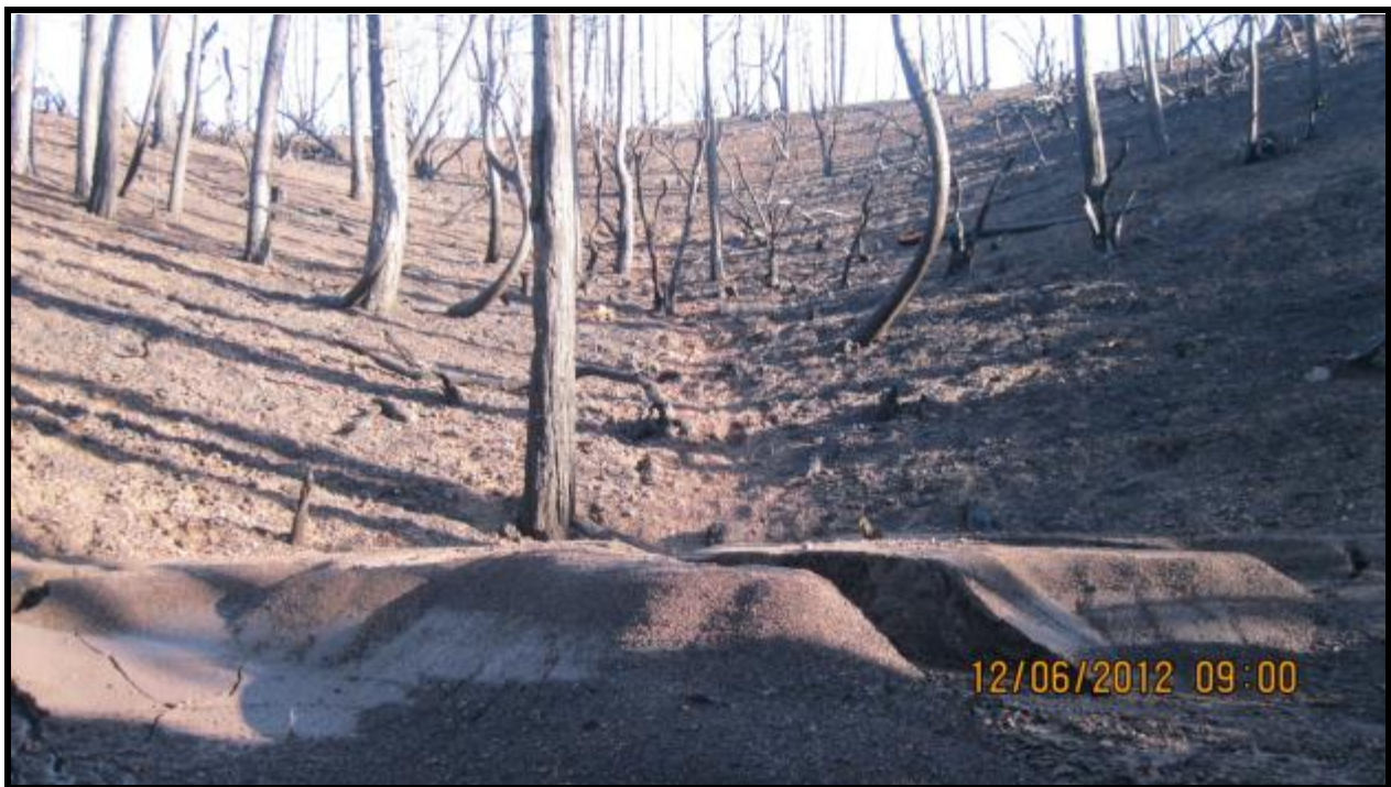
Figure 2. Depositional lobe at the front of fence #10. Channel incision is evident in the axis of the swale directly above the center of the deposit.
