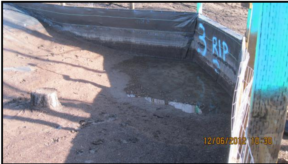
Figure 27. Sediment deposition in fence #3.
