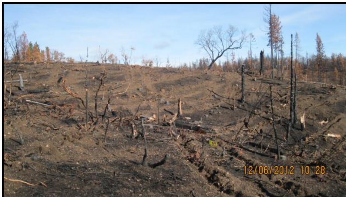
Figure 29. Contour ripping in the upper portion of the swale draining to fence #3.
