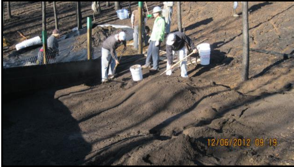
Figure 5. Laborers excavating sediment from fence #9.
